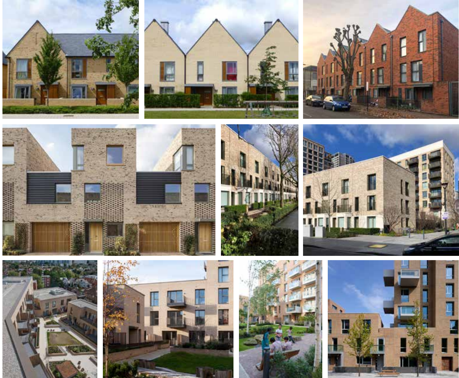
Right: Examples of high quality town centre family houses and apartments at a range of densities
